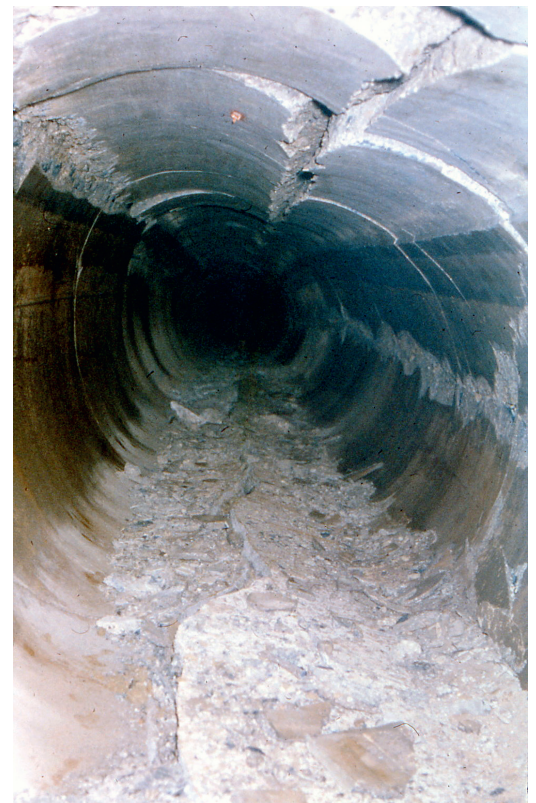
Fig. 3: a) Bending moment distribution and deformation of an originally circular (broken lines) support of a tunnel situated in the bedrock – landslide transition zone (shear zone) b) typical crack pattern of a tunnel support due to a landslide (the figure does not show the gallery described in this paper!) Photo: W. Eppensteiner
