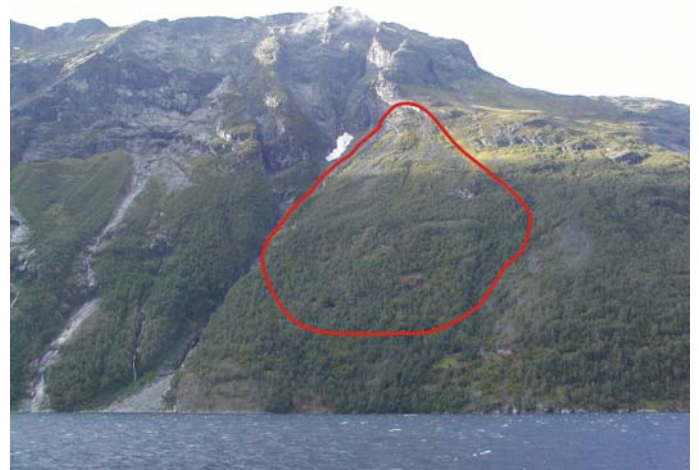
Figure 5. The Aknes rock slope. Unstable area marked by dashed line. Photo: Th. Sausgruber
